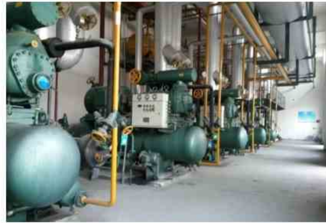
氨制冷系统 Ammonia Refrigeration System
