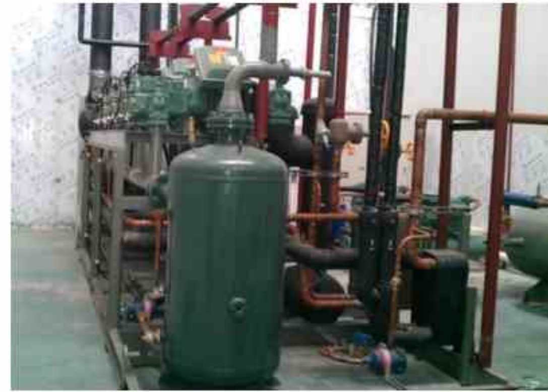
单机双级低温螺杆并联机组 Compound Two Stage Low-temperature Screw Compressor Unit
