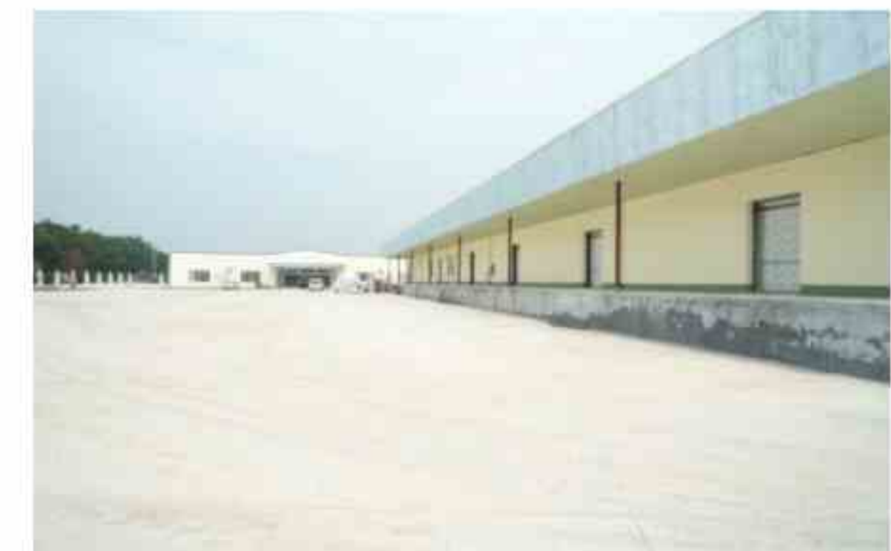
冷库 Cold Storage Room
